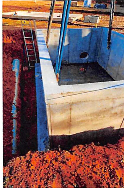
Figure 2- Vault Installation
