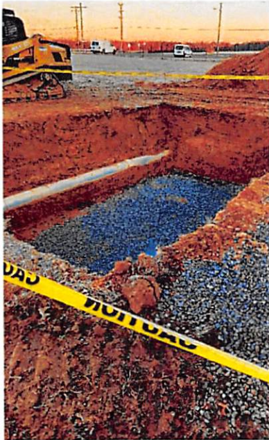
Figure 1- Vault Valve Excavation and preparation
